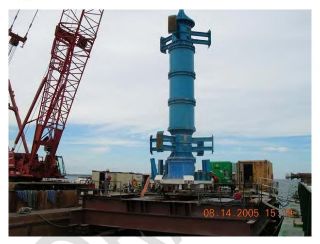
A 15-foot-diameter drill casing is then lowered inside the 18-foot conductor casing and reaches from the top of the sea bed down into the rock to form a seal.
