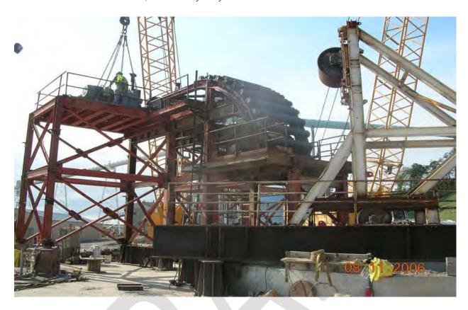
The TBM would begin boring operations, with the excavated material conveyed behind and vertically up the drop shaft to another horizontal conveyor belt, where it would be trucked away from the intake area:
